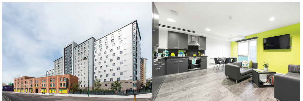
Photos: Shared kitchen / living area, exterior of Crescent House.
